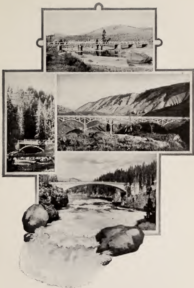
GROUP OF PARK BRIDGES.
